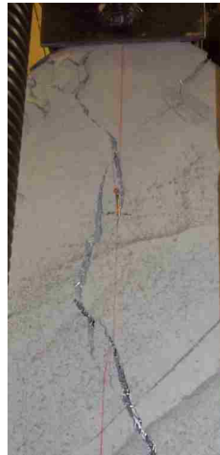
(b) Crack through face of wallette.
