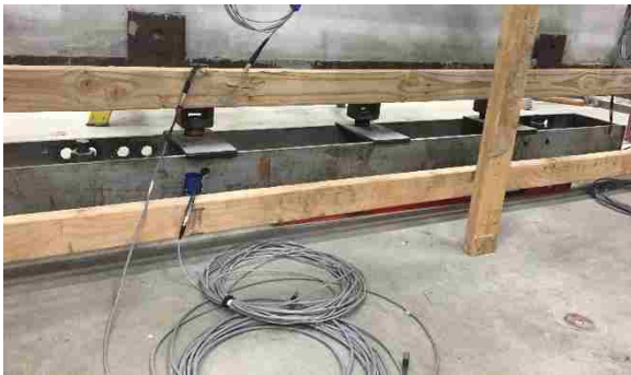
(c) Clevises attached to bottom of wall channel.
