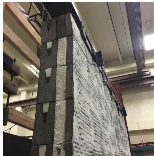
(b) Crack through top course.
