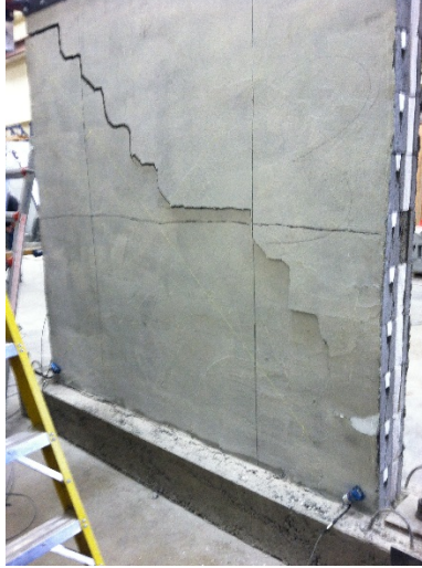
(b) Diagonal crack.
