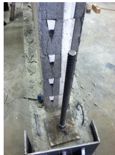
(c) Cracking in webs.
