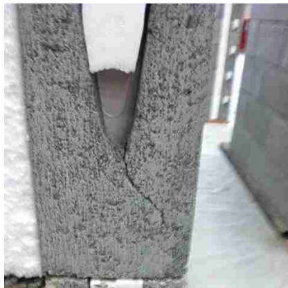
(a) Crack in block prior to testing.
