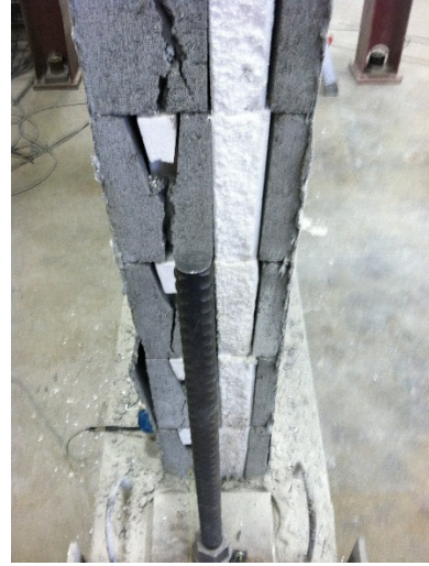
(c) Cracks through webs.
