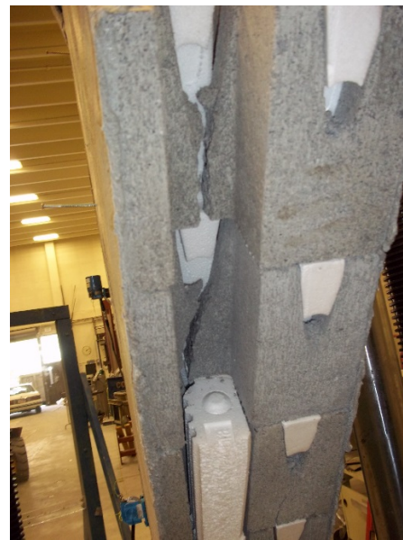
(b) Cracking through webs.
