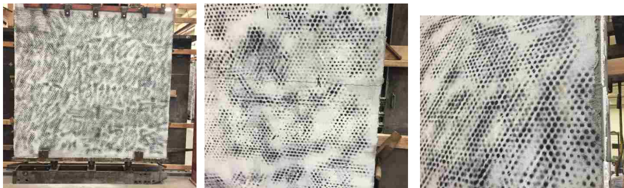
(a) Overall appearance. (b) Crack below third point (c) Crack at top of wall.
