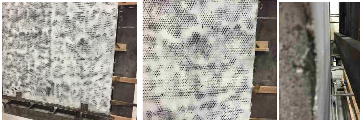
(a) Overall view.
