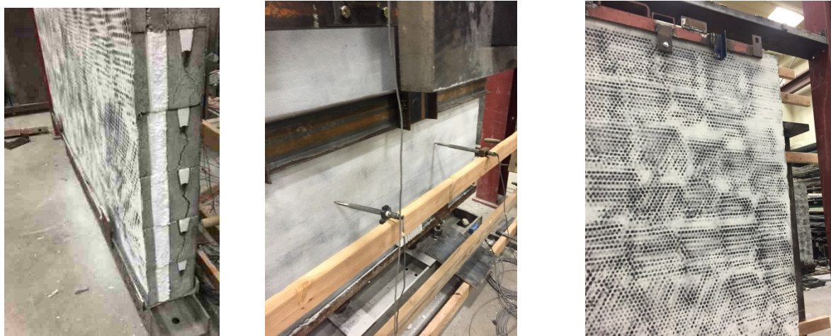
(a) Cracking in webs. (b) Cracking at bottom of wall. (c) No visible cracks in top of wall.
