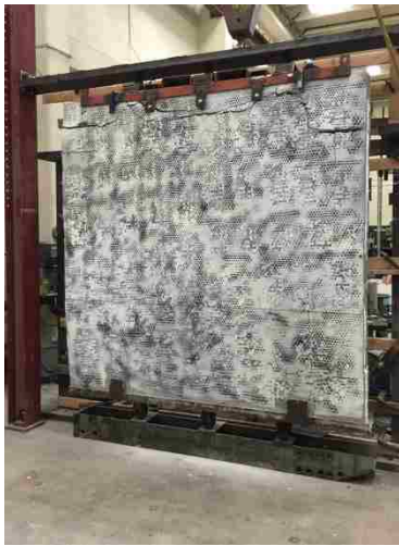
(a) Overall view
