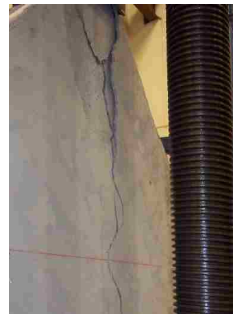
(c) Crack on face.
