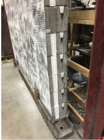
(a) Cracks in webs.
